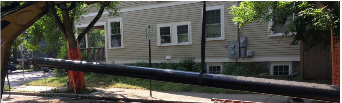
Figure 10. Plastic pipe replacement in Brookline, Massachusetts.
